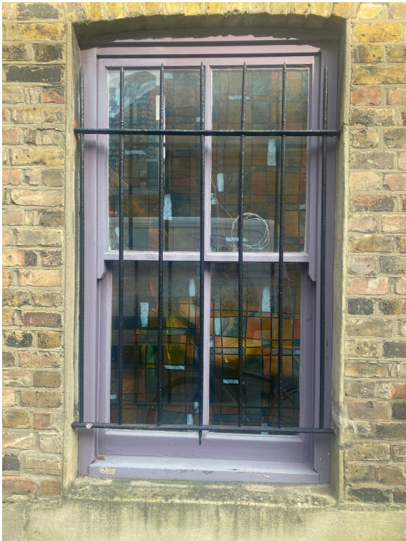
South-facing ground floor window
